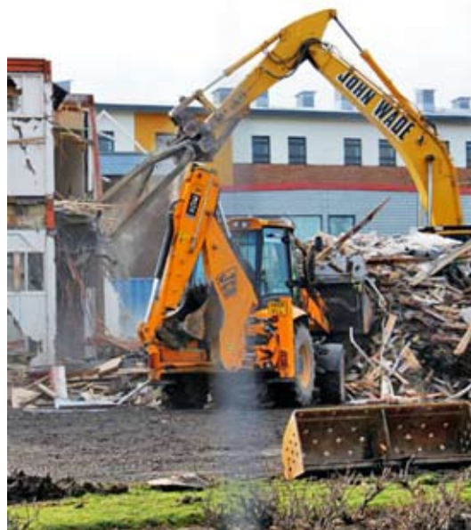
The final stage of demolition at the college.
