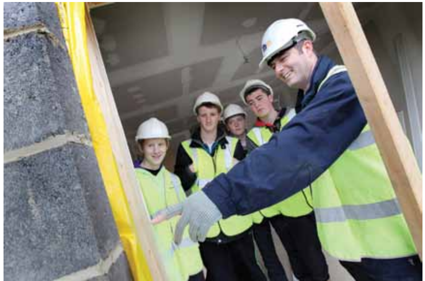
FHM Site Manager Martin Robson shows the Bishop Auckland College students around one of the apartments currently being built at Park Avenue Court, in Crook.
